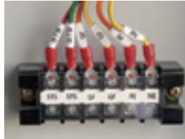
*Terminal board for remote control
